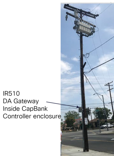
Figure 150 IR510 Overhead Line Installation
