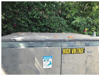
Figure 151 IR510 Underground Line Installation
